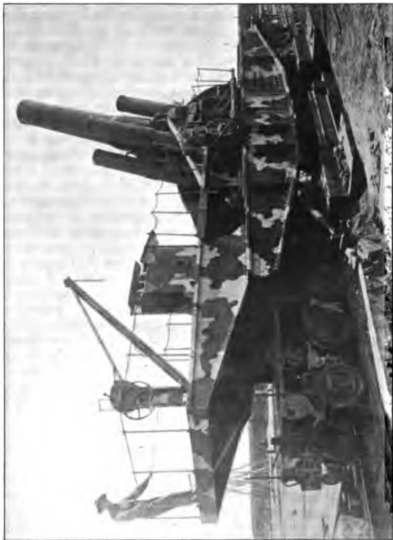
16-INCH AMERICAN HOWITZER MOUNT, MODEL 1918 (EMPLACED FOR HIGH ANGLE FIRING).
